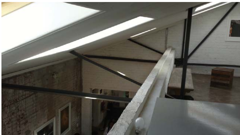
Figure 128 showing roof lighting in a multi-level studio in Arts on Main (Author 2012)
