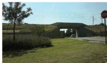
B showing a Gautrain Bridge over Antwerp Street going towards the Historical Village
