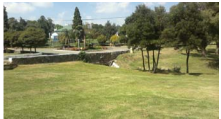
C Figure 103 showing the view of the bridge on Christies Hill (Author 2012)
