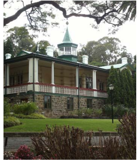
Figure 28 showing the Franz Hoenig Haus. The house was built for the first factory manager in 1896 and is now a historic house museum (Author 2012)
