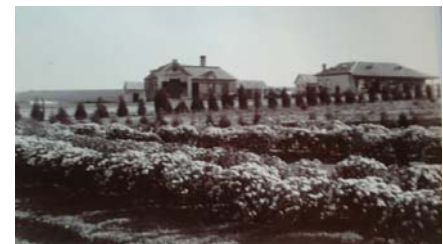
Figure 61 Photograph showing early tree planting in the Modderfontein village in the 1890s (Photograph from the Dynamite Company Museum Archive)
