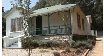
Figure 43 showing an original house (Author 2012)
