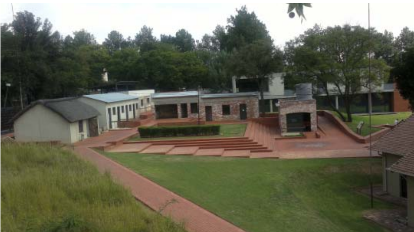
Figure 118 showing Liliesleaf, with moulding of the landscape into various platforms, steps, grass areas and ramps (Author 2012)
