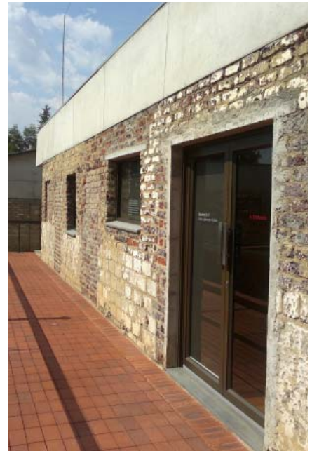
Figure 117 showing the existing old structure with new concrete additions at the Liliesleaf Liberation Centre (Author 2012)
