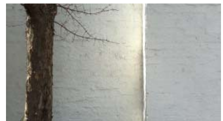
Figure 185 showing the bagged brick wall of a house on the corner of Roper and Anderson Street in Brooklyn, Pretoria (Author 2012)
