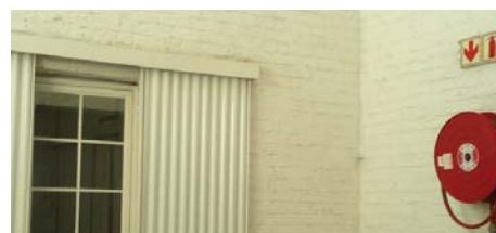
Figure 129 showing the use of corrugated iron and white painted facebrick in Arts on Main (Author 2012)
