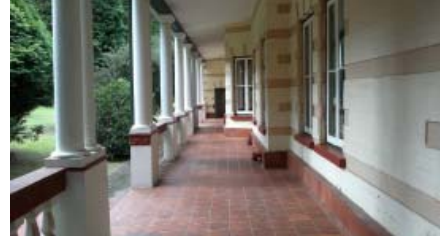
Figure 22 showing the veranda of the Franz Hoenig Haus with concrete columns instead of the original timber (Author 2012)
