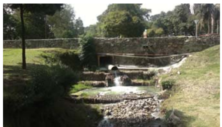
D Figure 106 showing the view of the bridge and river (Author 2012)
