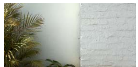
Figure 186 showing the mix of bagged and plastered wall of a house on the corner of Roper and Anderson Street in Brooklyn, Pretoria (Author 2012)
