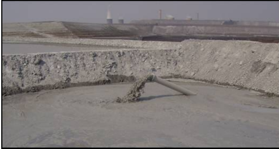
Figure 2.2 Deposition of fine ash-brine slurry onto a Fine Ash Dam
