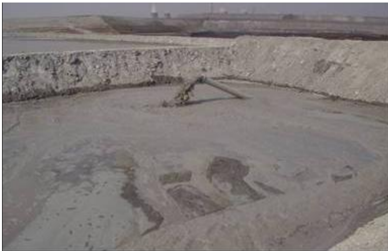
Figure 4.1 Deposition of slurry onto a FAD
