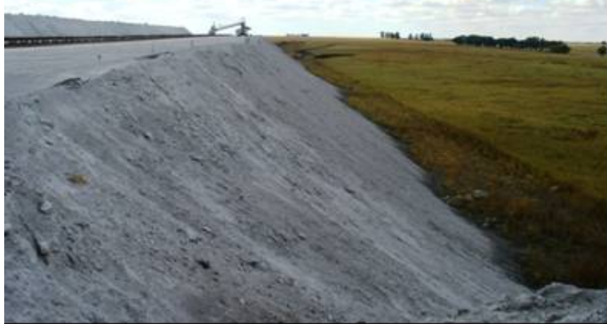
Figure 2.3 Disposal of dry fly ash at ESKOM's Tutuka plant
