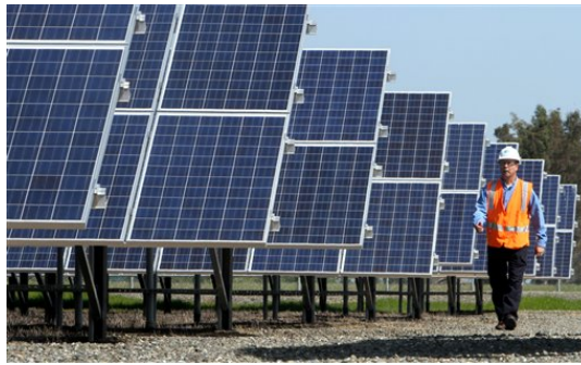
Figure 2.2: Field of Solar Collectors [8]
