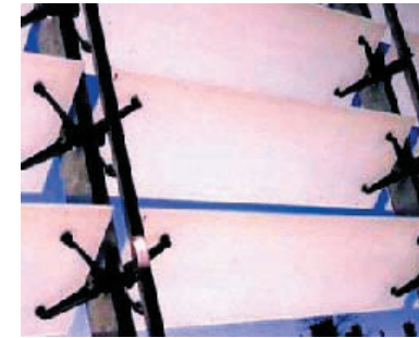
FIG. 4.3.6 External louvres prevent excessive heating and act as light-shelves
