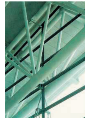
FIG. 4.4.11 "B" truss with sandwiched glazing
