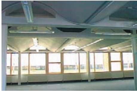
FIG. 4.3.4 Interior view of office space with shaped ceilings that aid in the thermal control systems of the building.
