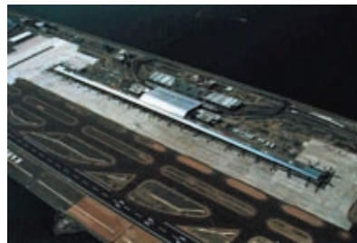
FIG. 4.4.2 Aerial view of Kansai Airport
