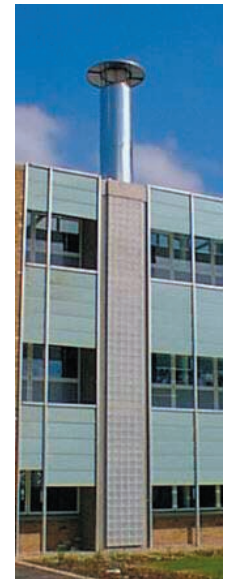
FIG. 4.3.3 Glass-fronted ventilation shafts to warm the air inside and create stack-effect
