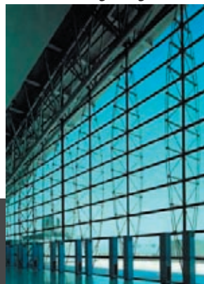
FIG.4.4.12 internal view of glazed gable wall
