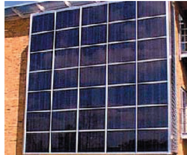
FIG. 4.3.5 Photovoltaic array on Southern facade of building (northern hemisphere)
