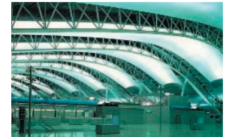
FIG. 4.4.4 Internal image of airport building
