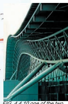
FIG. 4.4.10 one of the two great glazed gable walls
