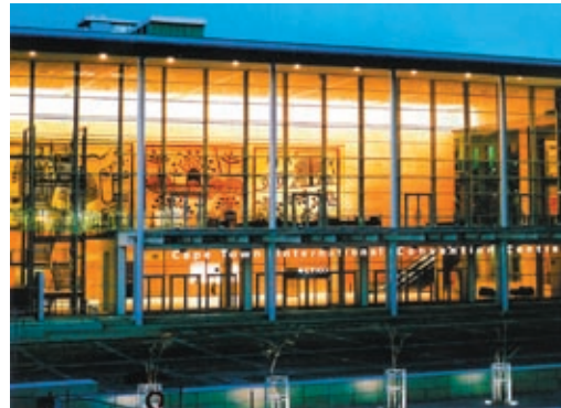
FIG. 4.5.2 entrance foyer from the exterior
