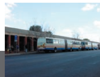
FIG 2.3.3 Existing regional bus facility at Pretoria Station
