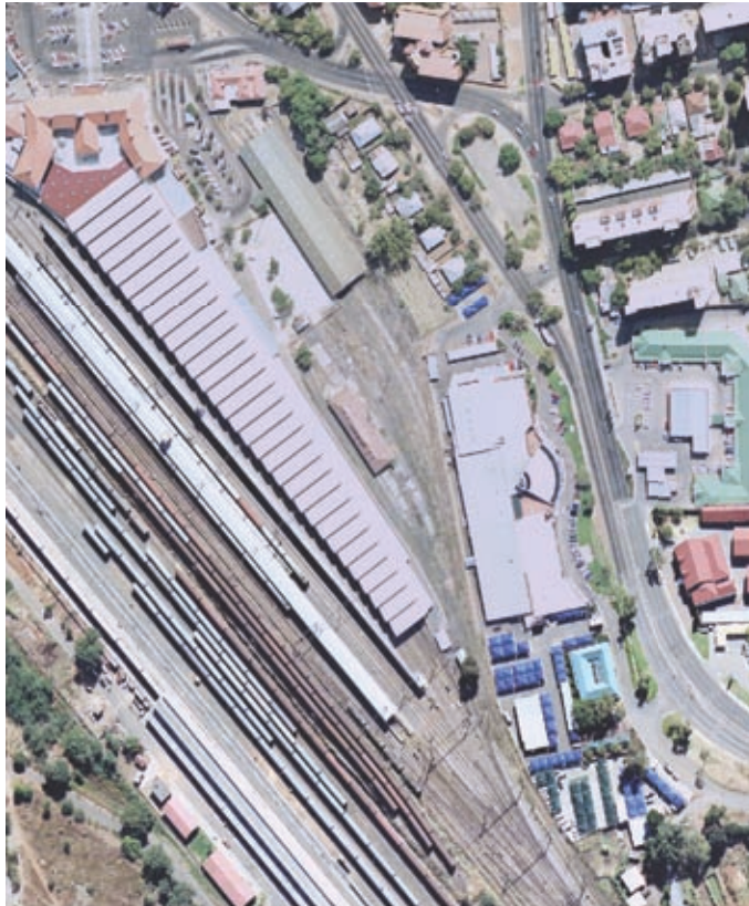
FIG. 2.7.7.1 Existing Landuse of site: Commercial motor vehicle showroom due for demolition with Gautrain Development. Existing landuse of precinct: abandoned Railway yard
