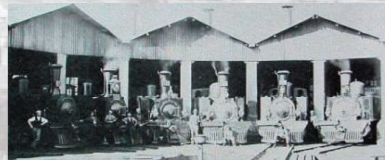
FIG. 1.5.17 Roundhouse at Waterval-Onder, circa 1895. The Pretoria roundhouse and this one were identical
