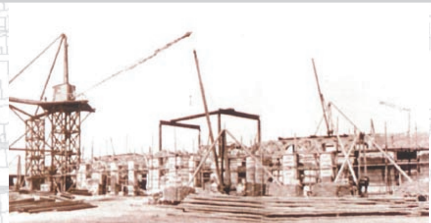
FIG. 1.5.21 The Pretoria Station under early construction - 1910
