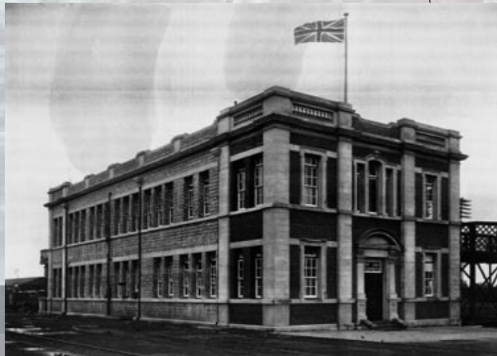
FIG. 1.5.15 CSAR Chief Mechanical Engineers Office, completed 1909, just west of Koch St alignment. Note the pedestrian bridge that connects the stair
