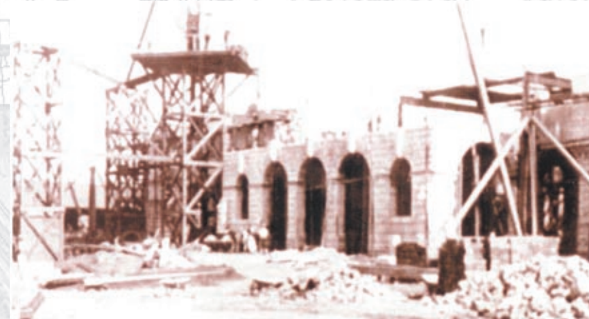
FIG. 1.5.22 The Pretoria Station under early construction - 1910
