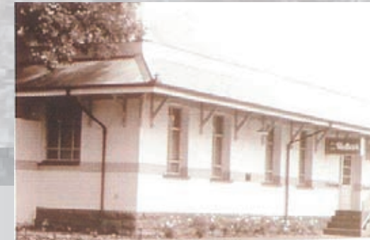
FIG. 1.5.14 Historical Signalling and Telegraph building occupied by Westbank
