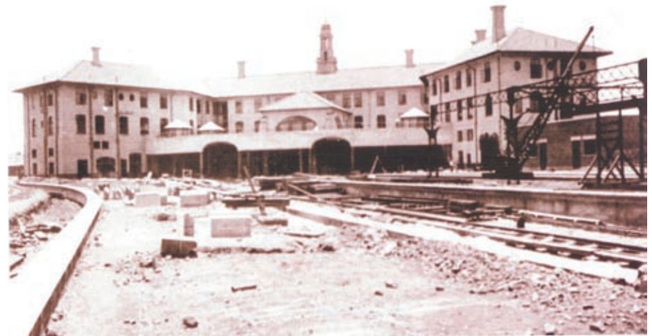
FIG. 1.5.9 A rare view of the south side of the Station building taken during construction in 1910
