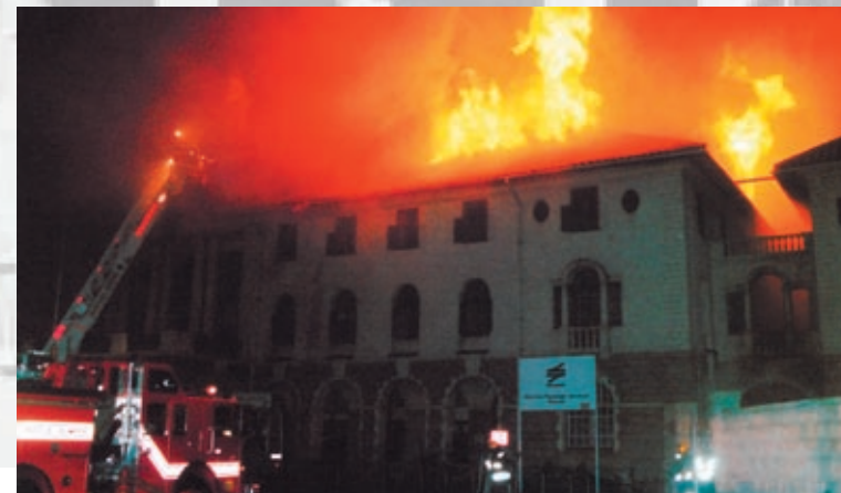
FIG. 1.5.10 Image of Pretoria Station during the blaze that almost destroyed the building in 2001
