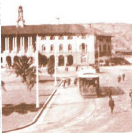
FIG. 1.5.25 A tram arrives at the Station along Market Street prior to 1925
