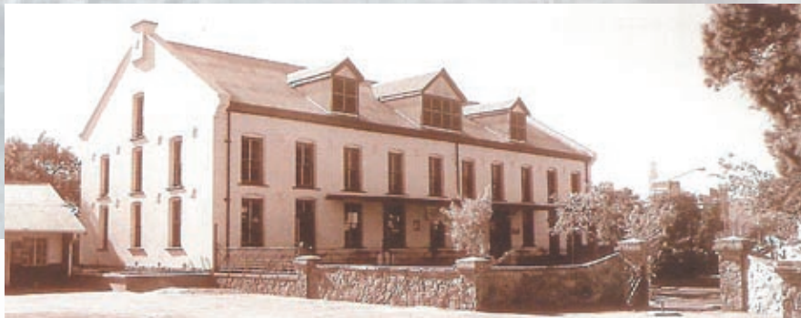
FIG. 1.5.11 Original NZASM Printing Store built in 1896. Currently used as Intersite offices
