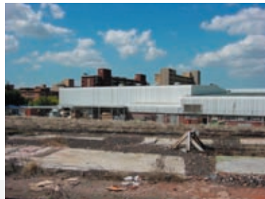
FIG. 1.4.20 Remains of demolished structures
