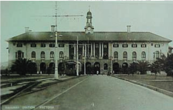
FIG. 1.5.23 CSAR Pretoria Station by Baker, completed in 1914
