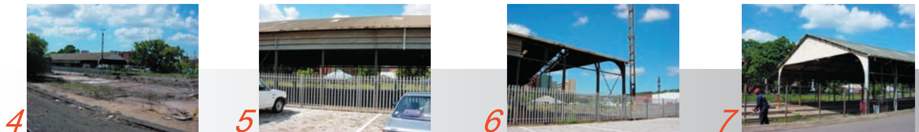
FIG.'s 1.4.4 - 7 CSAR Coach Washing Shed made from NZASM rails as roof supports, built 1904-10
