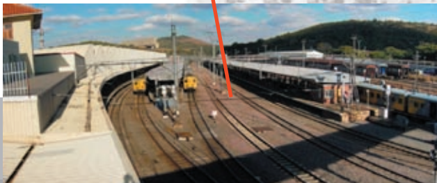
FIG. 1.3.17 View south east over the rail reserve
