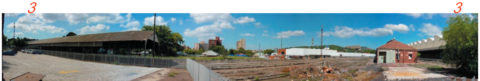
FIG. 1.4.3 Panoramic view north of site
