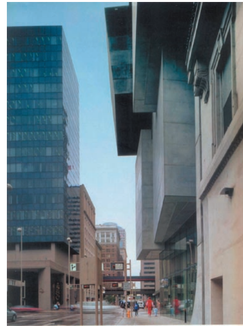
Figure 5-7 Concrete outcropping above the sidewalk (Halbe 2003)
