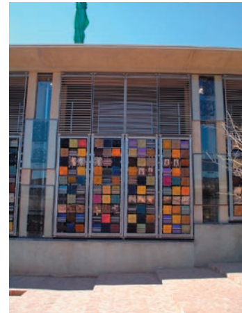
Figure 5-4 Decorative sun-screen panels on Western Facade (Roos, 2004)
