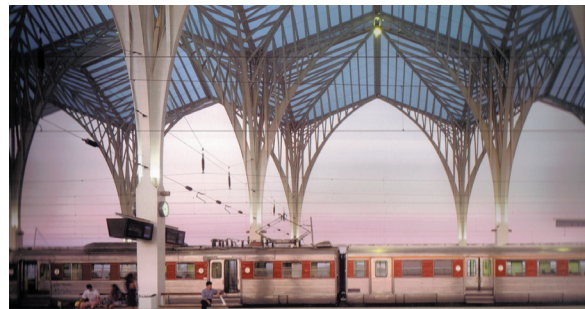
6.4 Left: Santiago Calatrava's Oriente Station, Lisbon, Portugal
