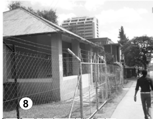
Figure 52 - north view along van der Walt Street.
