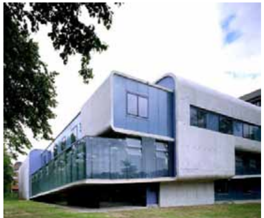
Figure 8 - ramp to first floor, NMR Laboratory, Utrecht.
