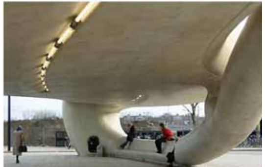
Figure 205 - image of application of GRP's in the Bus Station, Hoofddorp, Netherlands by NIO Architects 2003.
