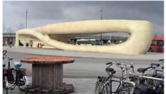
Figure 204 - image of application of GRP's in the Bus Station, Hoofddorp, Netherlands by NIO Architects 2003.
