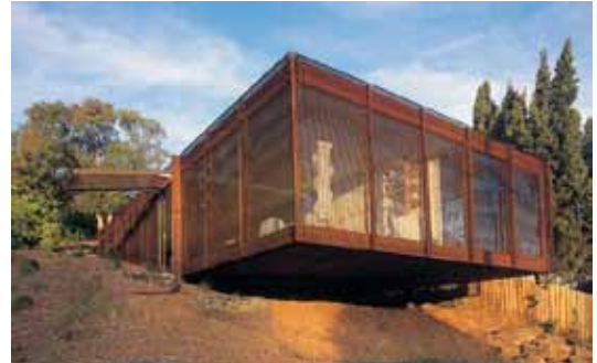
Figure 214 - image of similar stainless steel cladding used in Kew House, Melbourne, Australia by Sean Godsell 1996-1997.
