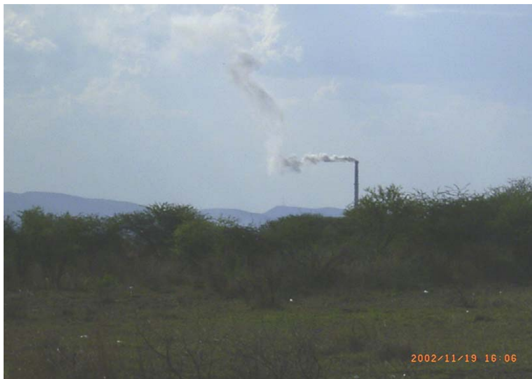
Figure 4.16: Example of Smelter emissions (North West Ecoforum, 2002).
