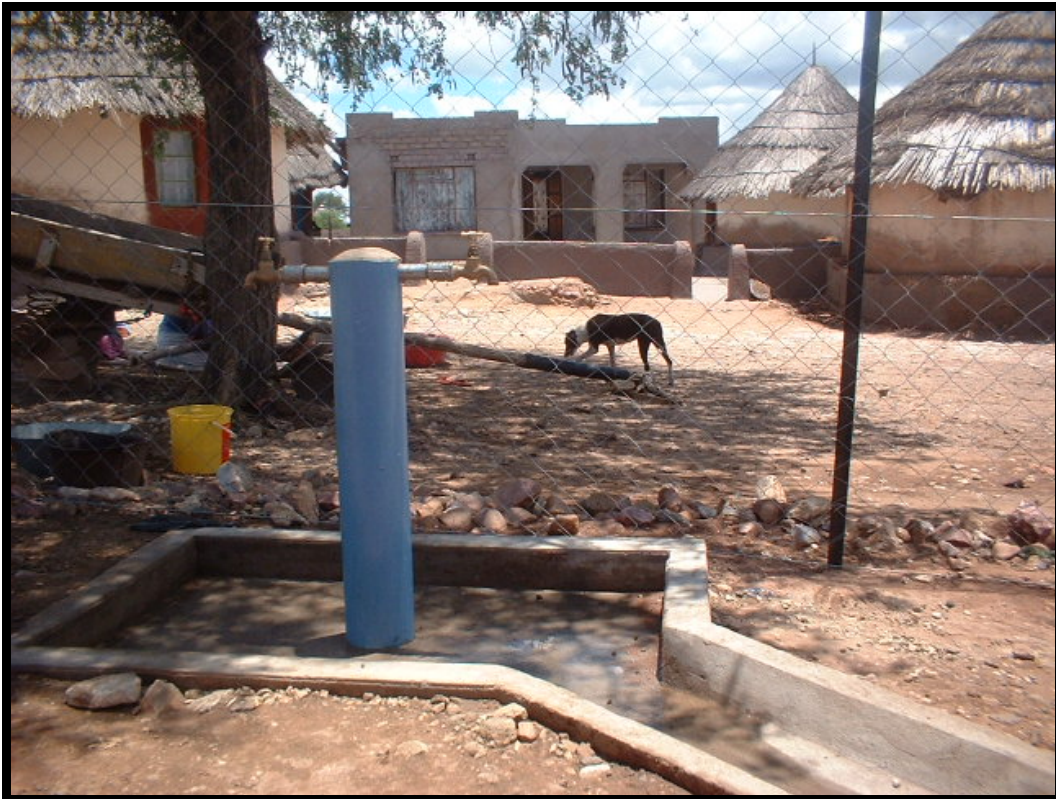
Figure 3.2: Typical communal taps used by rural households in village 1 in the Vhembe region of the Limpopo Province, South Africa
