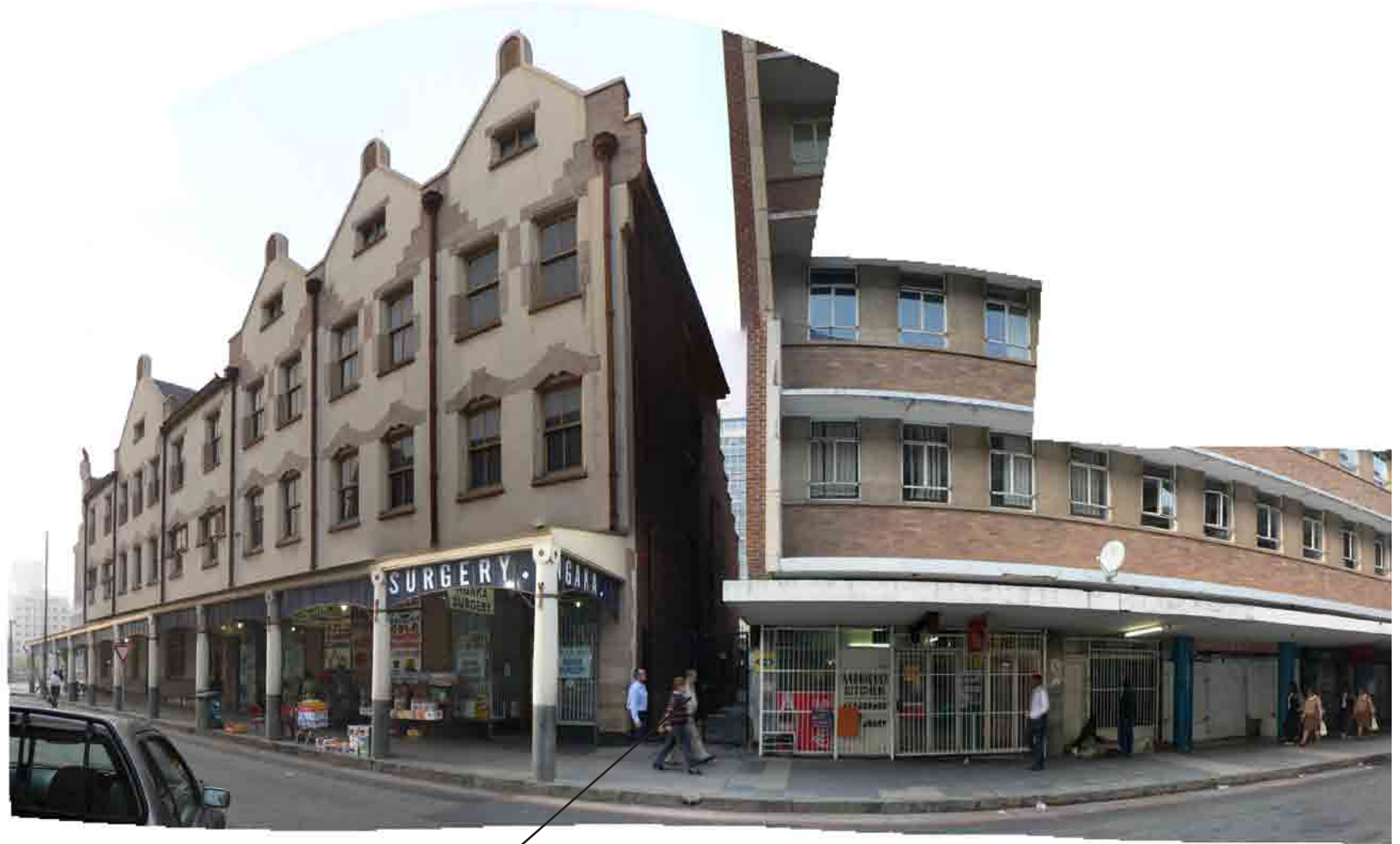
▲ Fig. 254 Photograph of site
