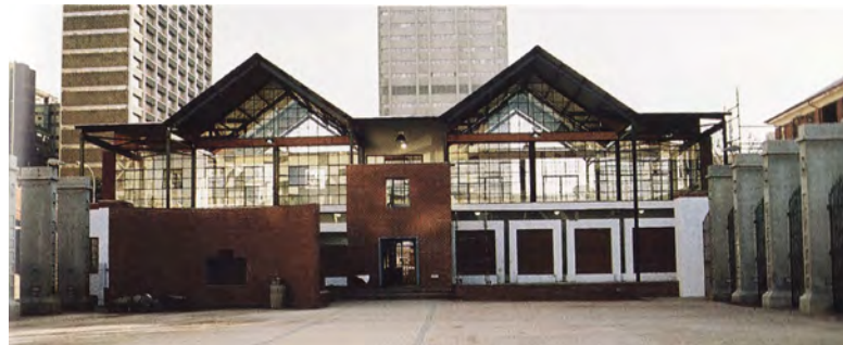
[Fig. 43] Reinterpretation of the original roof, supported on lightweight steel and glass construction
