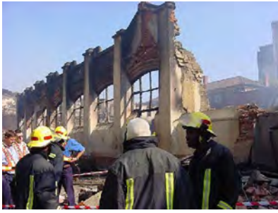
[Fig. 45] Firemen inspect the damage from the fire.
