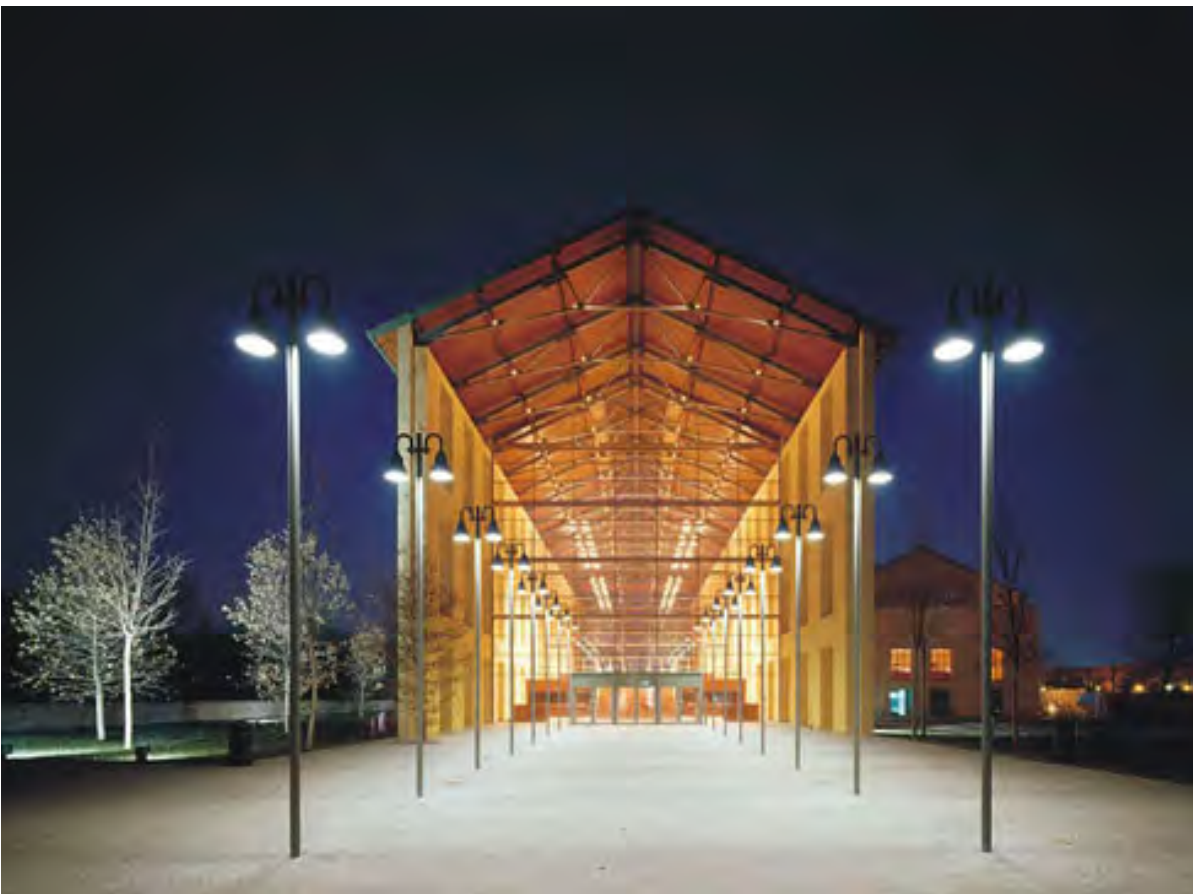
[Fig. 39] Showing glass curtain wall which allow an undisturbed view of the volume of the building
