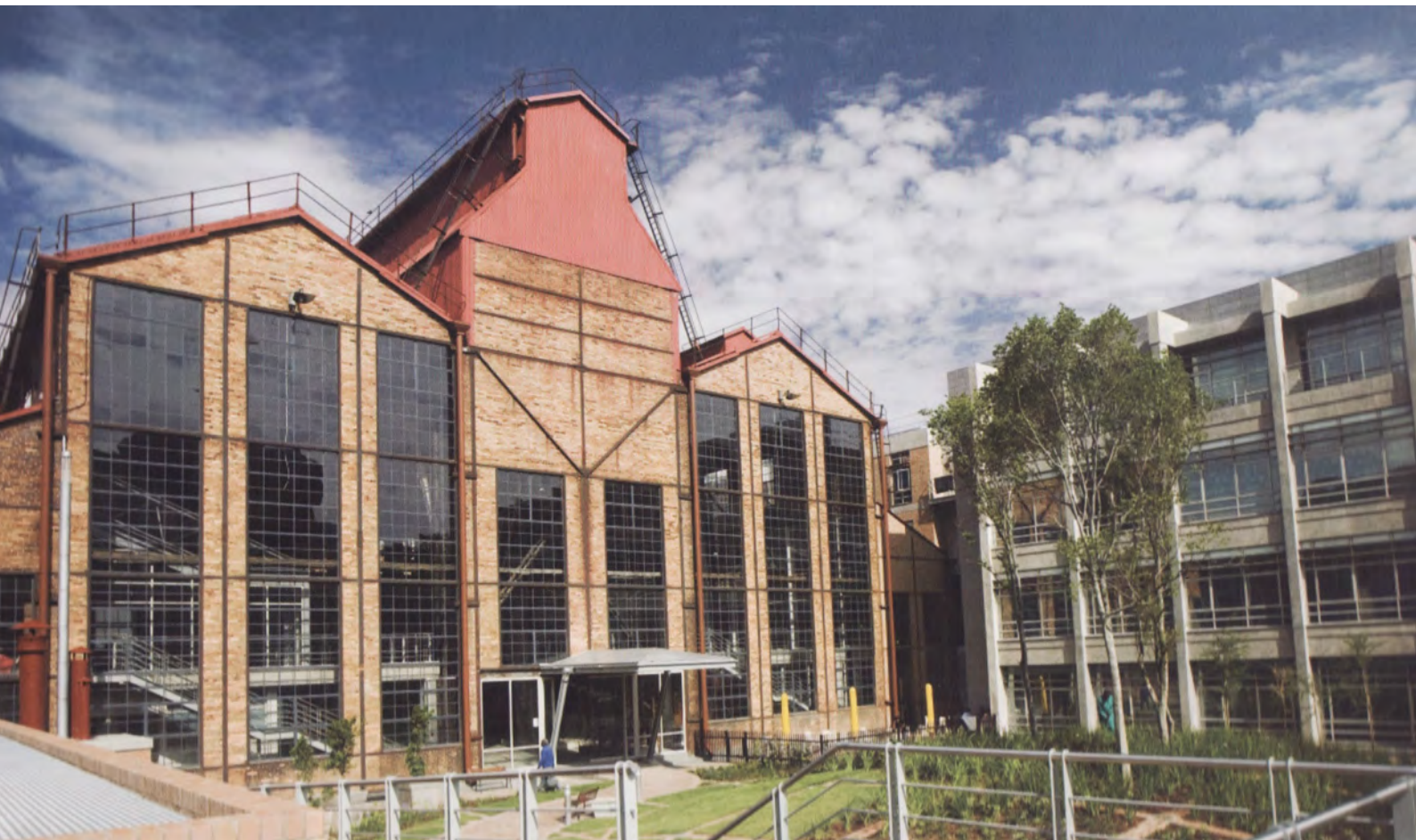
[Fig. 50] View of the refurbished South Boiler House (left), and the new office building (right) from turbine square
