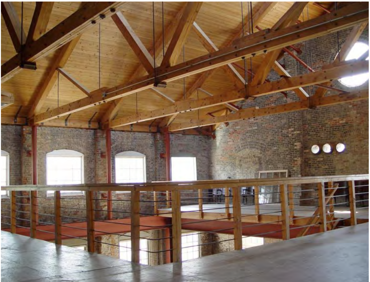
[Fig. 35] Showing the clear contrast between the existing brickwork and the new timber and red steel.
