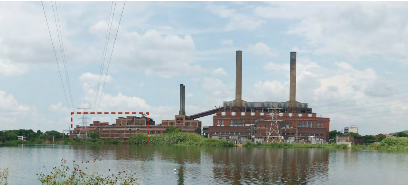
[Fig. 12] Photograph of how the power station looks today, highlighting the old part of the plant that is shown in the historical photograph (fig. 13), one can see how much the plant has grown over the years.
