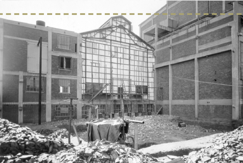
[Fig. 104] Excavation to prepare for the 1935 addition
