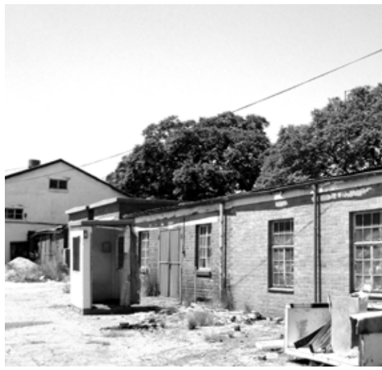
38. INTERNAL COURTYARD SPACE ON SITE (AUTHOR, 2010).
