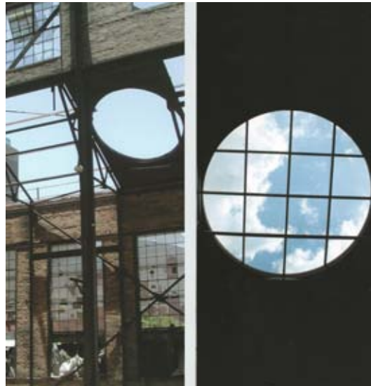
fig. 66_ Skylights were kept in place as memory of the old structure (TPSP Architects, 2008)
