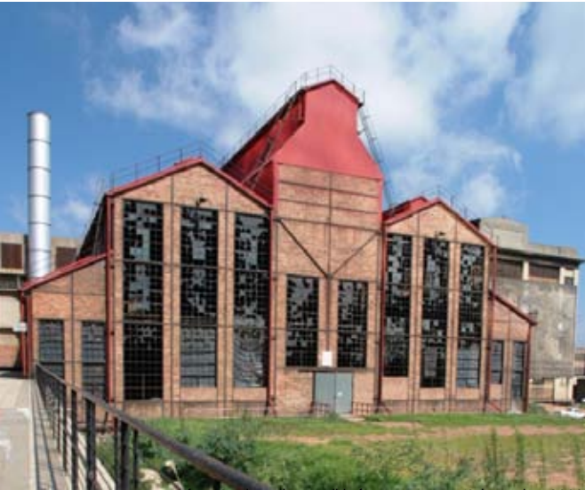
fig. 62_ The Turbine Hall before construction (Schoemaker, 2008)
