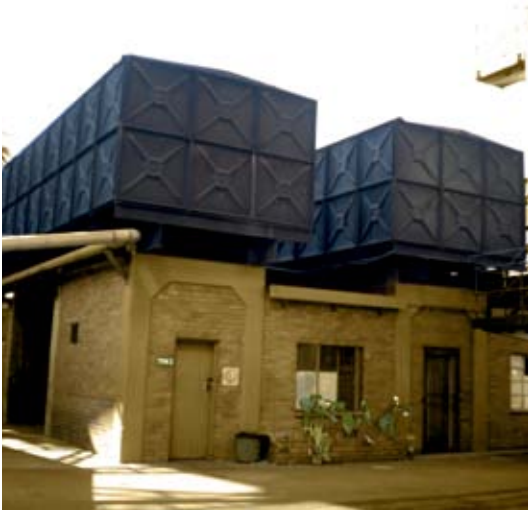
fig. 94_ Part of the steel oil tanks will be converted into water storage tanks
