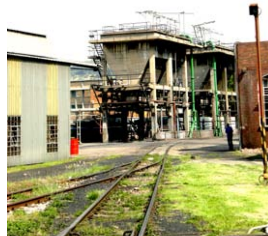
fig. 31_ View 3: Ash hoppers_after coal is burned it is taken here where contractors pick it up for use in for example concrete
