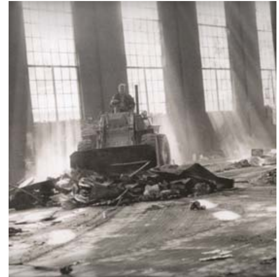
fig. 64_ The Turbine hall was cleaned out in 2000 and once again fenced of (Gaule, 2008)
