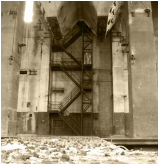
fig. 76_ Interior view of The Boiler House, photograph taken from the entrance of the building
