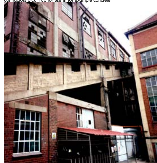
fig. 34_ View 6: Station A, some of the buildings on site has been decommissioned for over 60 years
