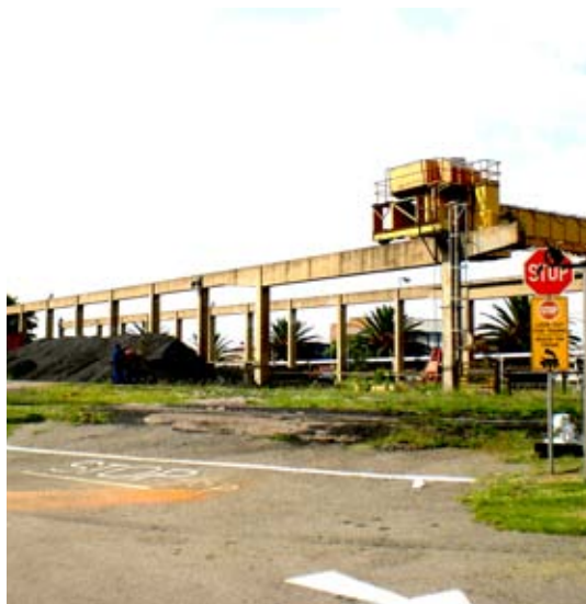
fig. 29_ View 1: The Coal bunkers_trains enter the site and dump the coal in the bunkers, from here it is taken to the fireboxes by conveyor
