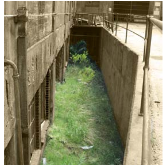
fig. 78_ The Northern facade of the Boiler House extends into the ground, and stand as a fort in the landscape
