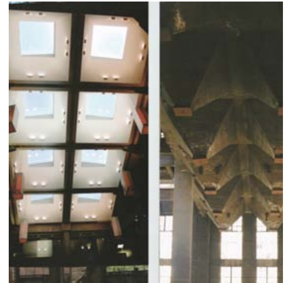
fig. 67_ The original concrete hoppers in the demolished North boiler house are commemorated as skylights in their original location (TPSP Architects, 2008)
