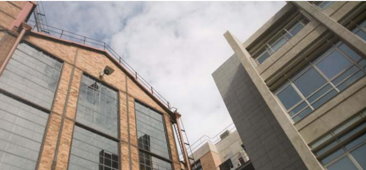
fig. 63_ The adapted Turbine Hall on the left with the new office structure on the right, the scale and material choice compliments the old structure (Tibler Group, 2008)
