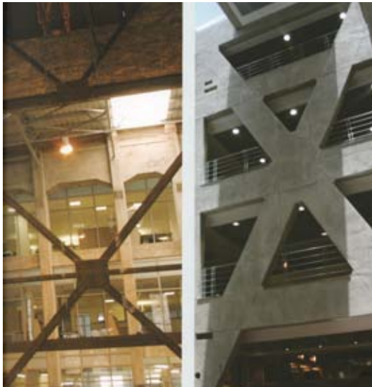
fig. 65_ The X-brace structure of the building was reinterpreted as structure and aesthetic device (TPSP Architects, 2008)
