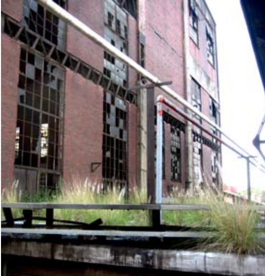
fig. 149_ The brick work of the dilapidated 1935 Boiler House will be reused to construct part of the showroom
