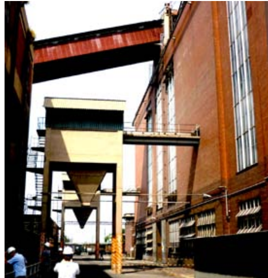
fig. 33_ View 5: Station A on the left and Station B on the right, with moth-balled ash hoppers in-between
