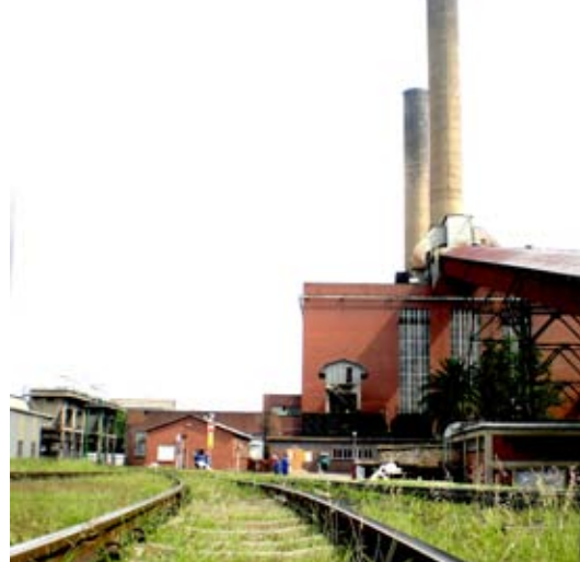
fig. 30_ View 2: Station B and the conveyor belt that takes coal from the coal bunkers to the fireboxes
