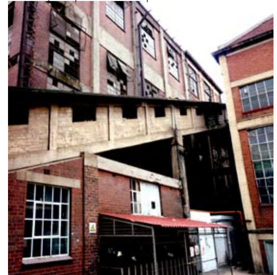
fig. 34_ View 6: Station A, some of the buildings on site has been decommissioned for over 60 years
