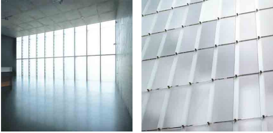
Fig. 7.29 and 7.30 Kunsthaus Bregenz, Austria, by Peter Zumthor. Overlapping panes of glass form a skylit glass wall in the lobby
