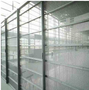
Fig. 7.31 Rovaniemi Airport terminal, Finland, by Heikkinen-Komonen. Steel Mesh screens shape spaces and defines routes.
