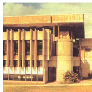
Fig. 7.41 Exterior of the Joint Christian Chapel, Dar Es Salaam, designed by Anthony B. Almeida
