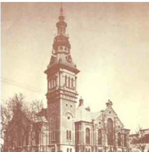
Fig. 3.5 Bosman Street Church, completed in 1905 on the corner of Bosman and Vermeulen streets. Declared a national monument.
