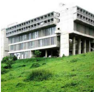
Fig. 2.56 The Dominican Monastery of Sainte-Marie-de-la-Tourette, designed by Le Corbusier
