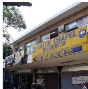
Fig. 3.24 Signage marking a church space in the inner city
