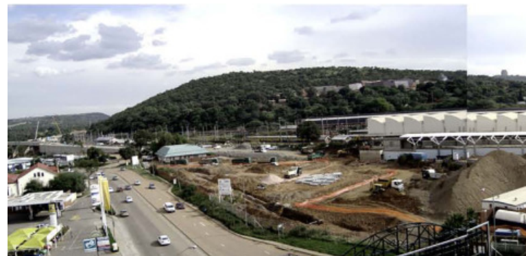
Figure 07. Panoramic view of the Station Precinct
