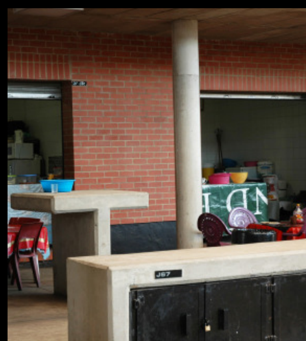
Figure 63. Internal view with pre-cast concrete furniture
