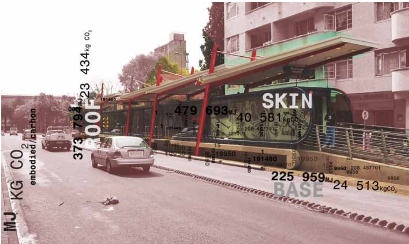
Figure 4-25: Embodied energy and carbon footprint of Rea Vaya Station [Source: Author]
