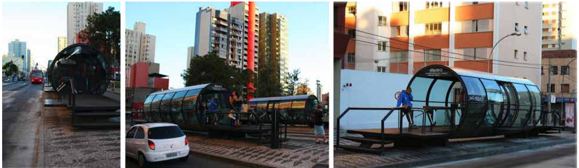
Figure 5-05: Placing of station on street edge [source: www.greatbuildings.com, accessed 14 March 2010 ]
