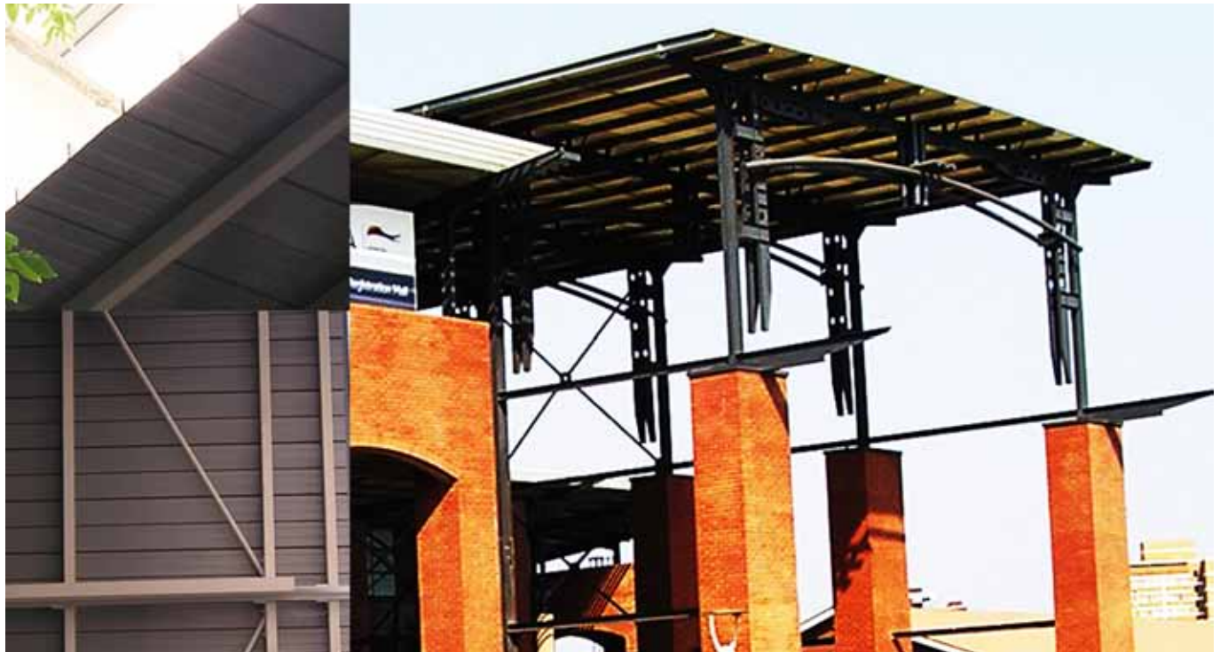
Figure 9-10: Brownbuilt roof sheeting fixed at a very high level. [Source: Author].
