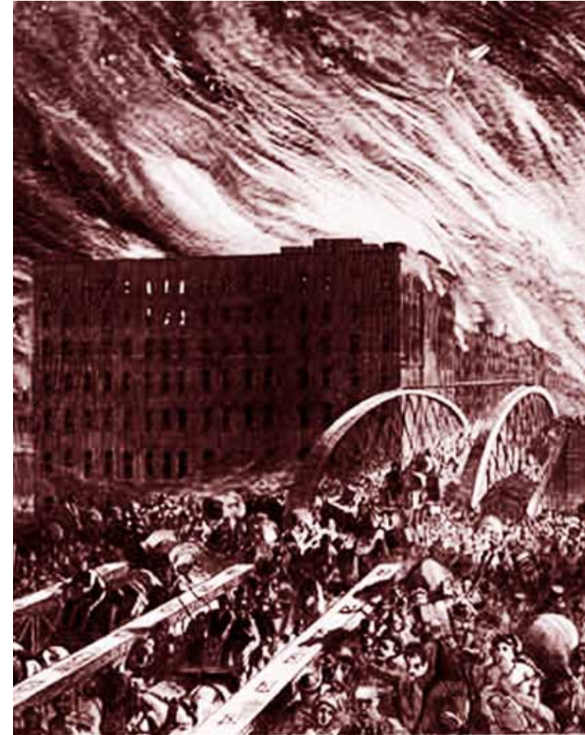
Figure 2-08: Heatwaves and increasing affect of fire ["The great Chicago Fire" - [ http://contentloco.com/travel/top-things-you-should-know-about-chicago.aspx ]
