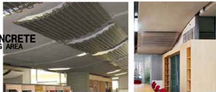
Figure 5-18: Ceiling detail [Source: Author]
