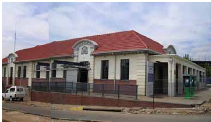
Figure 3-09: Entrance to Gautrain and Old Accounting building [Source: Author]
