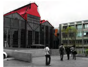
Turbine Square, Johannesburg, South Africa
