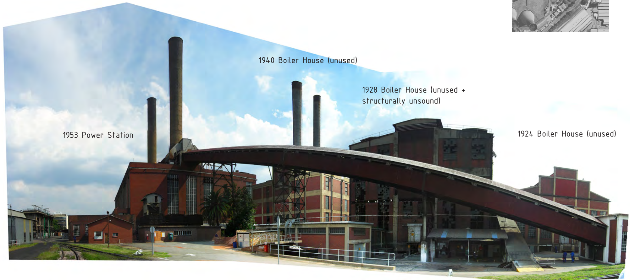
Fig 4.11 View of unused and current power station
