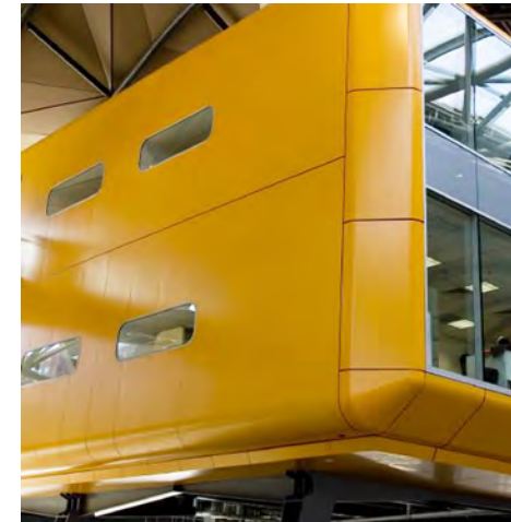
Fig 6.3 Structure of new building consists of steel frame with cladding, structure is hidden.
