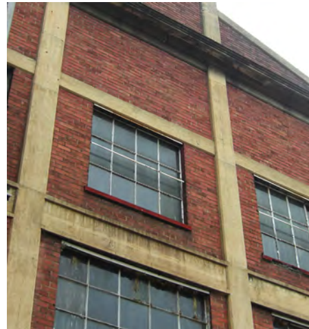
Fig 6.2 Structure of existing building consists of concrete frame with brick infill, structure is exposed.
