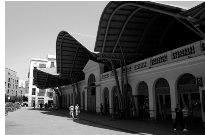
Fig 3.9 New roof over existing building.
