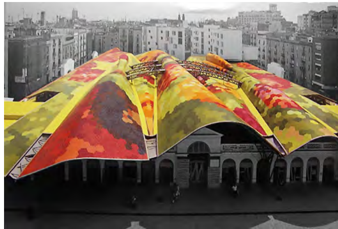
Fig 3.8 Roof of Santa Caterina Market and surrounding context.
