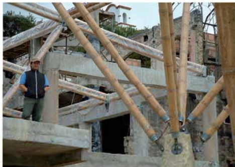
5. bamboo as structure column
