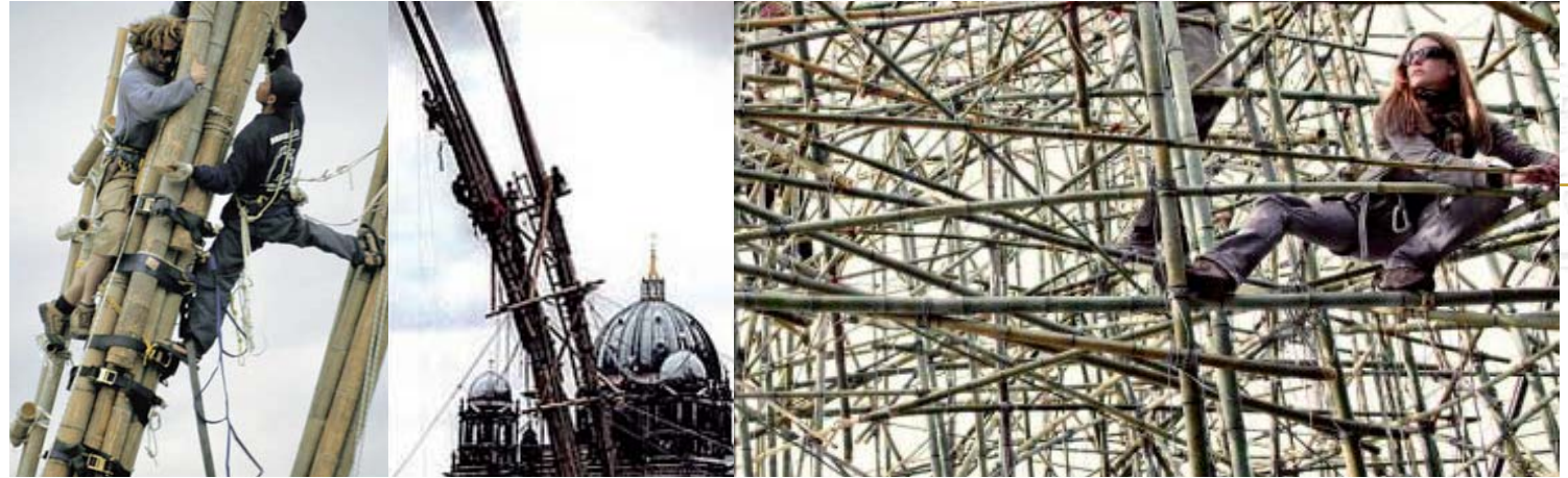
Figure 122, 123, 124: Live building workshop as testing ground for bamboo construction for South Africa.
