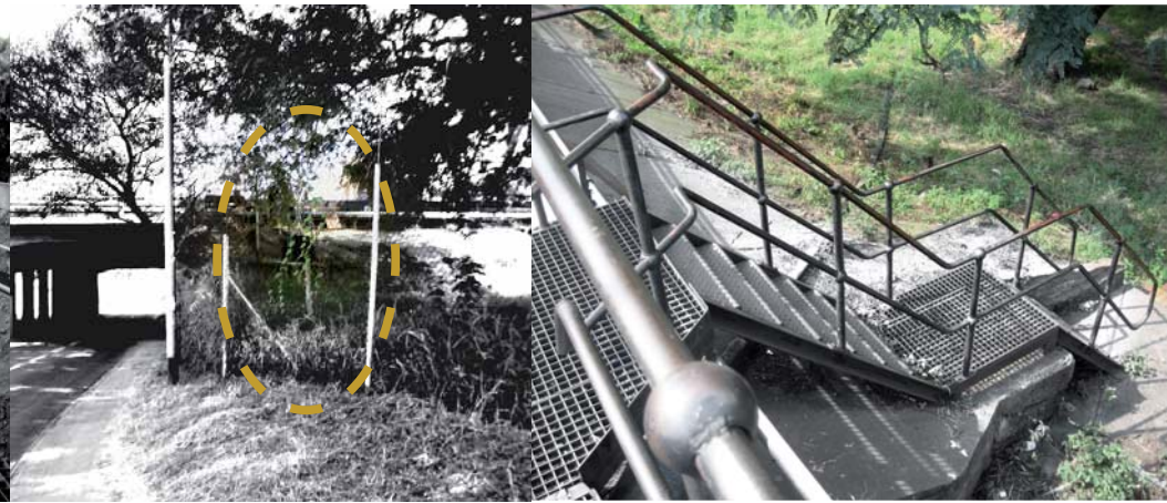
Figure 46,47 : Steel steps down to Buitekant Street
