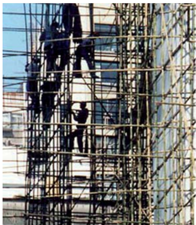
1. bamboo scaffolding & construction
