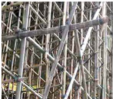
1. bamboo scaffolding & construction
