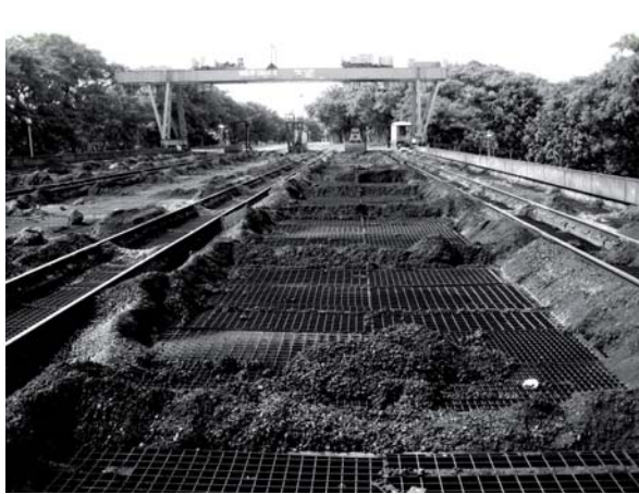
Figure 45 : On top of the bunker
