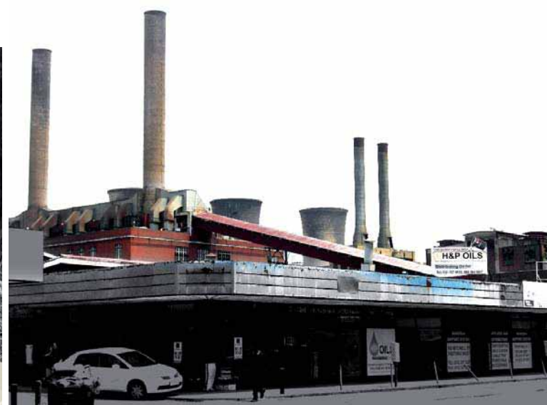
Figure 15e - Presence of the power station
