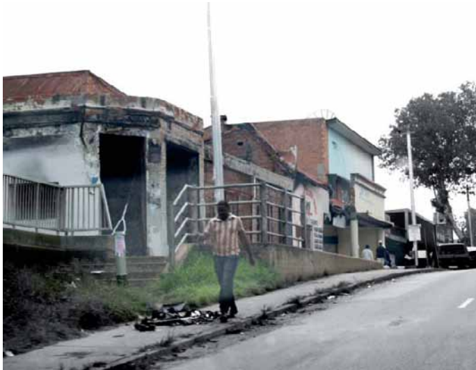
Figure 16d - Signs of dilapidation and neglect
