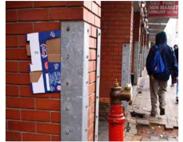
Figure 359: Protection of face brick edge, Metro Mall
