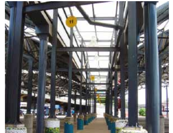
Figure 360: Framed and covered walkway at Faraday Market Transport Interchange
