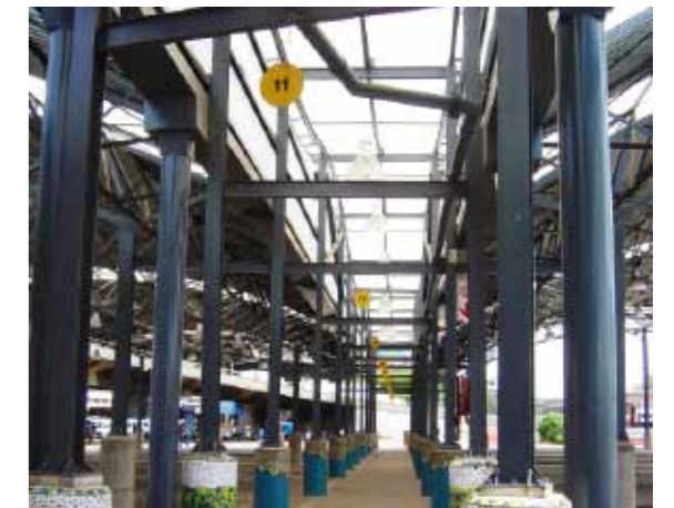
Figure 360: Framed and covered walkway at Faraday Market Transport Interchange
