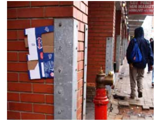
Figure 359: Protection of face brick edge, Metro Mall
