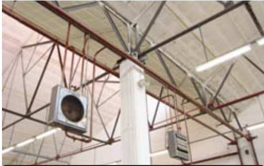
Figure 86. Existing ventilation system (Author, 2010).
