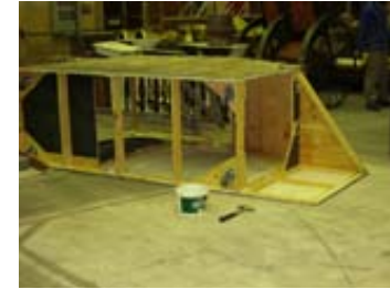
Figure 173. Construction of a rostra, Pretoria State Theatre (Author, 2010).
