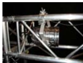
Figure 208. Floodlight temporarily attached to Z-Line truss (Author, 2010).
