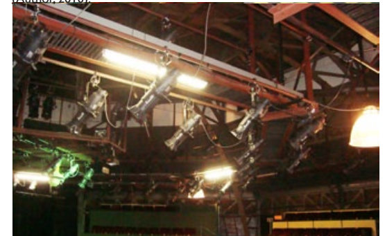
Figure 143. Lighting system in the Main Theatre fixed to the existing roof structure (Author, 2010).
