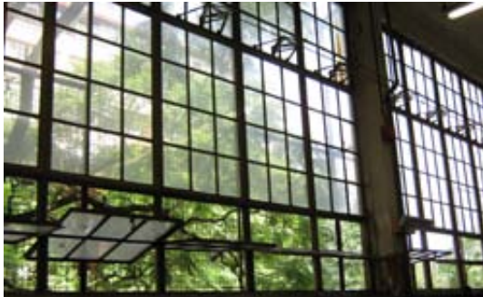
Figure 76. Steel frame windows in South Facade (Author,2010).
