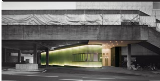
Figure 112. Exterior view of the Pop-Up Theatre (De Boer, 2009).
