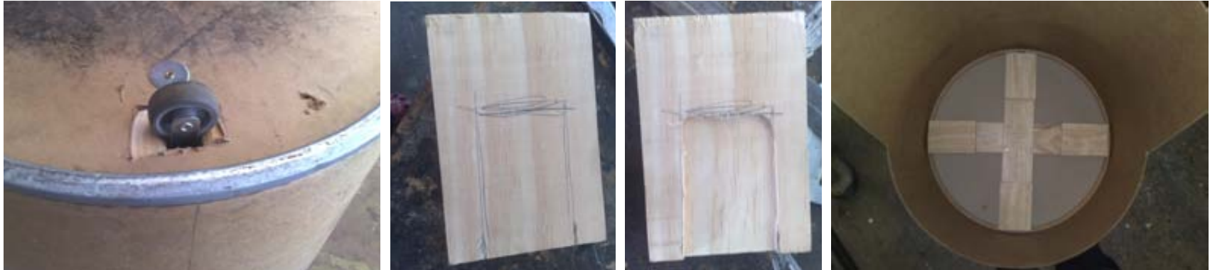
Figure 264. The wood members are fixed to the base of the drum with wood screws and washers. Four pieces of timber are cut to size and a groove is made in each, to fit over the connections of the casters. These pieces are then fixed over the casters and screwed to the wood underneath. This is done to secure the casters in place (Author,2010).
