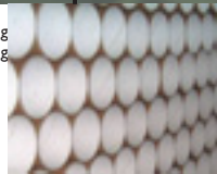
75ø Cardboard tubes fixed together with clear silicon in 270x270x270 cubes. Cubes are fixed to each other with 4ø threaded rod.
