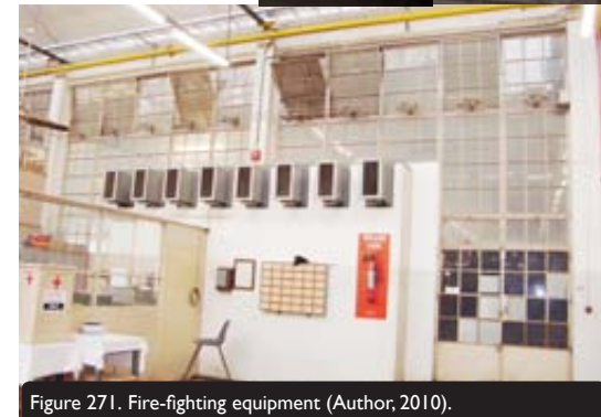
Figure 271. Fire-fighting equipment (Author, 2010).
