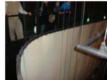
Figure 175. Canvas cyclorama suspended with cables, Johannesburg Theatre (Author, 2010).
