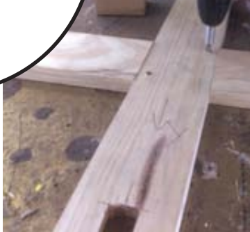
Figure 263. Two 38x114mm pieces of timber are cut to 600mm lengths. The ends are rounded and a slot is cut in each end for a casters to fit through. The two pieces are fixed together with a shiplap joint and secured with wood-glue and wood-screws .A caster is placed in each slot and fixed to the wood with wood-screws. Matching holes are cut in the base of the drum to accommodate the casters. The assembly is placed in the bottom of the drum (Author,2010).
