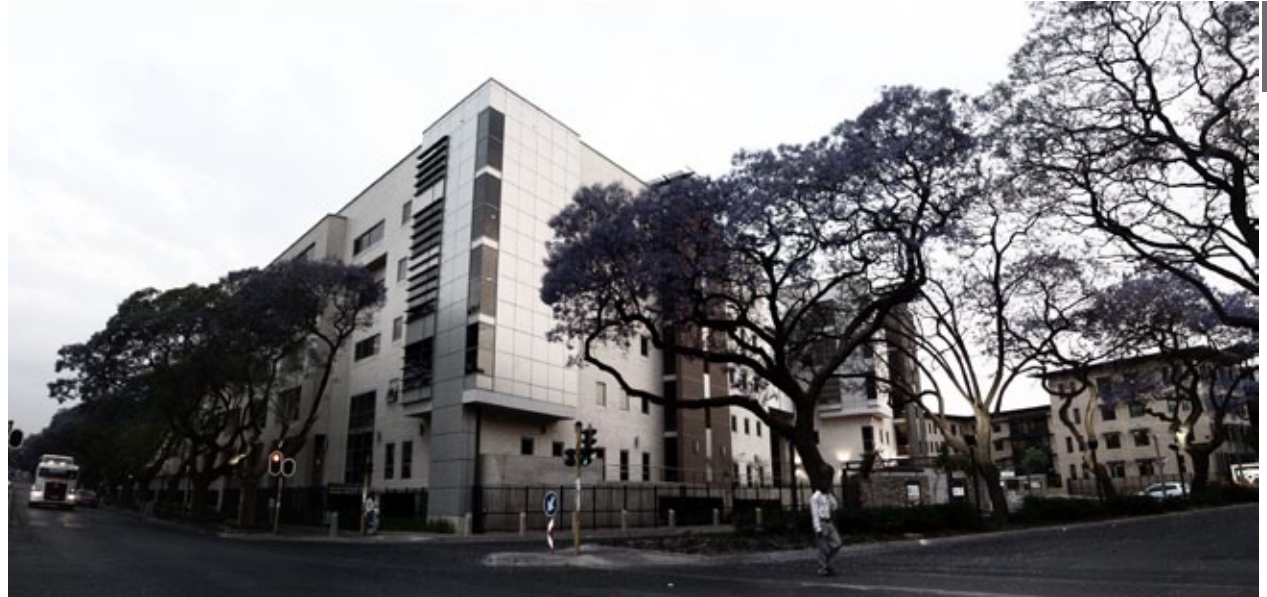
Fig. 1.3 Department of Minerals and Energy An Invaluable opportunity has been missed to engage with the pedestrianised street edge. The building is impenetrable on street level, which makes it a non-negotiable to the passer by. In invaluable opportunity to engage with the quieter street and adjacent open corner in the foreground has been missed.
