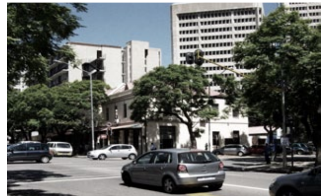
Fig. 3.19 Panagos Building, opposite Jewish Synagogue on Paul Kruger Street
