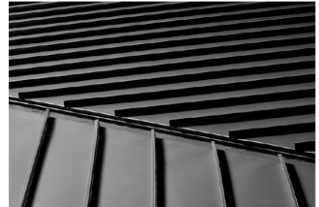
Fig. 7.12 Standing seam roof finish ( http://lgcroofingnj.com )
