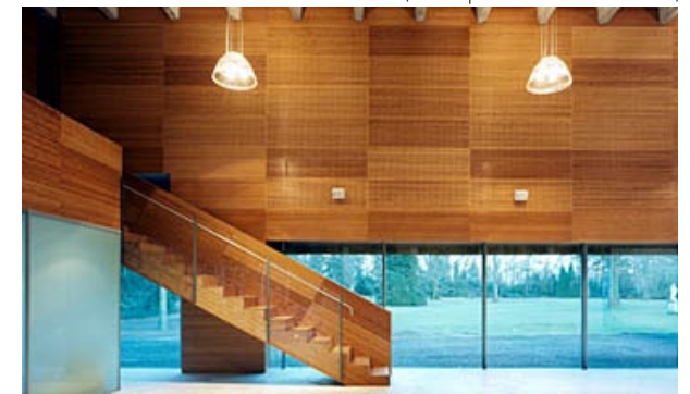
Fig. 7.31 Showing laminated bamboo cladding ( www.pandabamboo.co.za )
