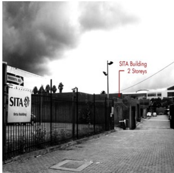
Fig. 4.8 Photo by Author Showing the view of the Existing SITA Building From Proes Street
