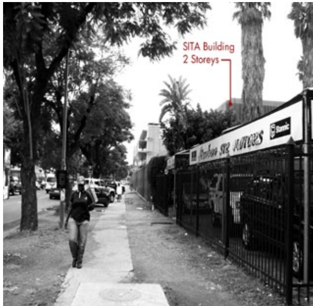
Fig. 4.7 Photo by Author Showing the view of the Existing SITA Building from the corner of Paul Kruger and Struben Street
