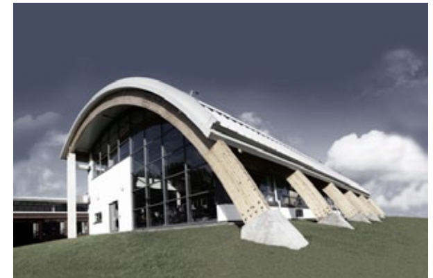
Fig. 7.13 Standing seam roof finish ( http://www.euroclad.com )
