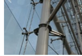
Fig. 7.15-7.17 Showing the Rose Centre at the Museum of Natural history in New York. This transparent building has a very high curtain wall supported by a tensioned stainless steel system similar to the system employed within this project.
