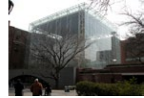
Fig. 7.15-7.17 Showing the Rose Centre at the Museum of Natural history in New York. This transparent building has a very high curtain wall supported by a tensioned stainless steel system similar to the system employed within this project.
