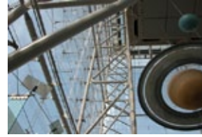
Fig. 7.15-7.17 Showing the Rose Centre at the Museum of Natural history in New York. This transparent building has a very high curtain wall supported by a tensioned stainless steel system similar to the system employed within this project.
