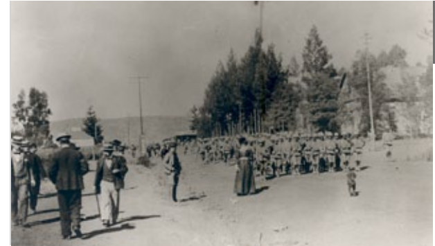
Fig. 3.17 One of the First Photo's of Paul Kruger Street
