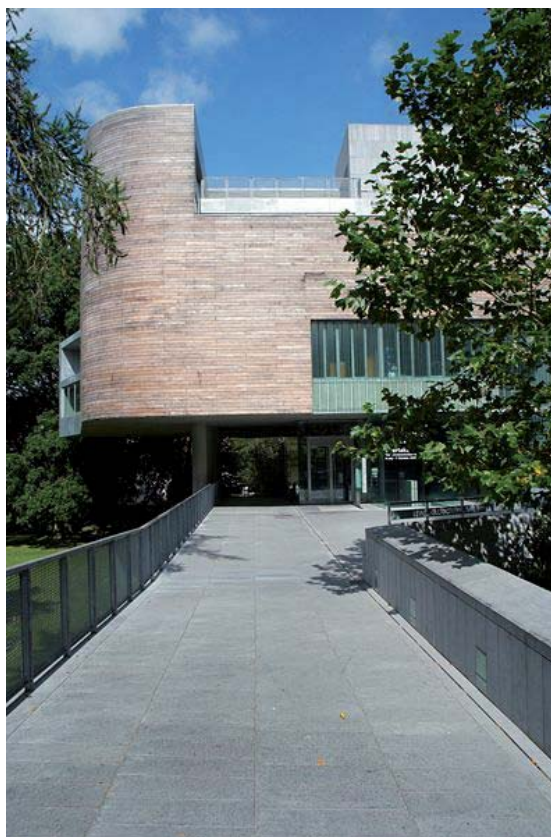
FIG 4.4_Access route onto the building's 'podium'
