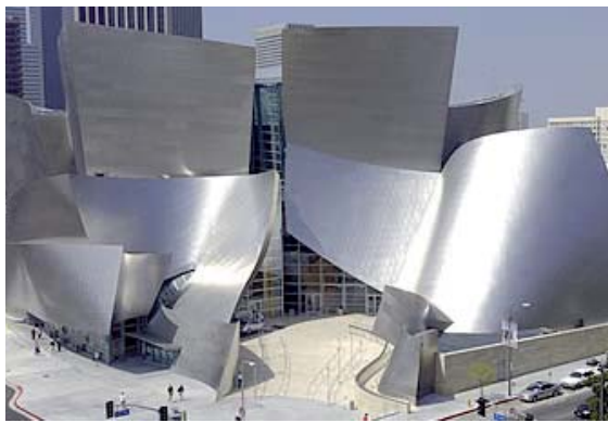
FIG 4.7_ Exterior stainless steel cladding
