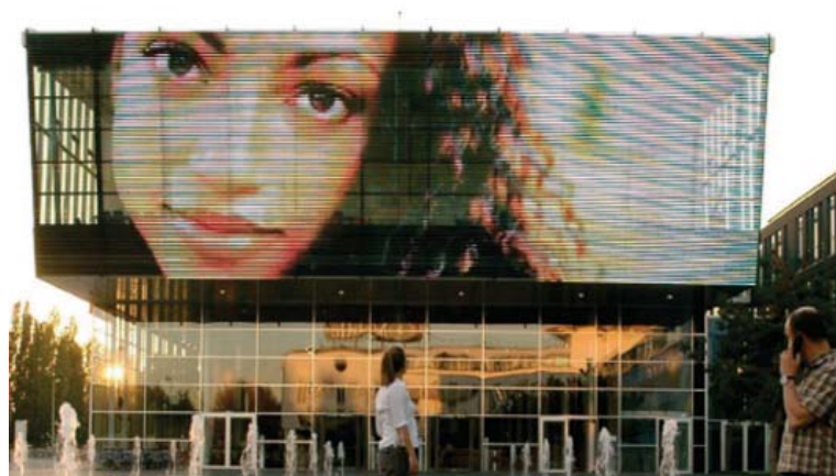
FIG 3.4_Mediamesh creates multimedia experience on building facade
