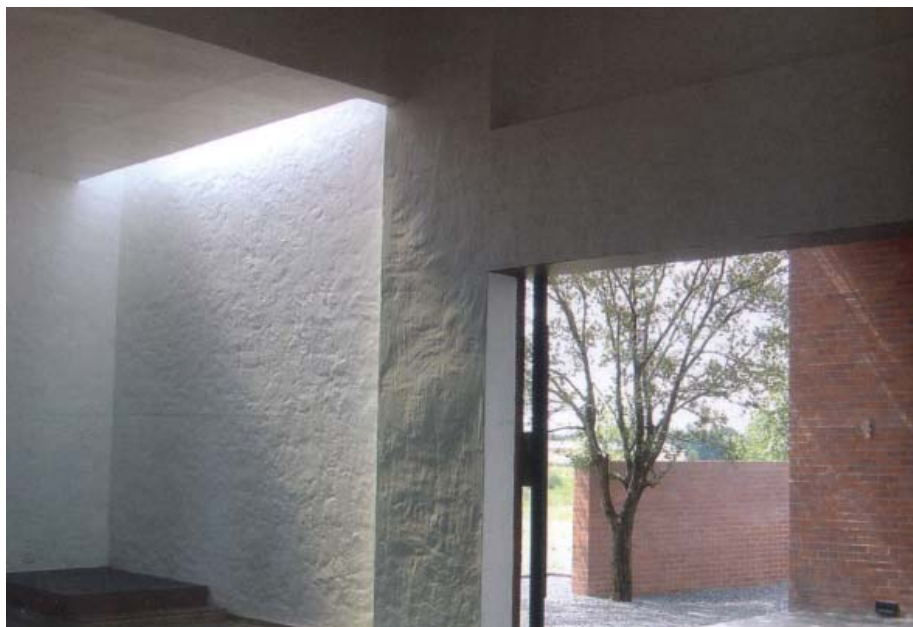
FIG 3.10_Skylight used to provide soft natural light in the creation of a sense of tranquility
