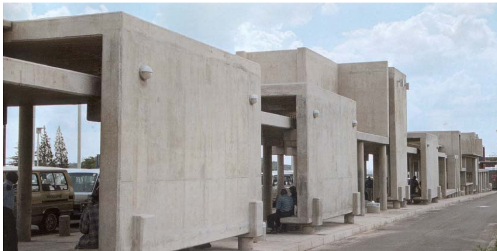
FIG 3.29_Massing provides shelter and gives a sense of security and safety
