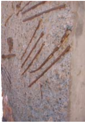
Figure 101. Objects embedded in concrete (Theart, 2007)
