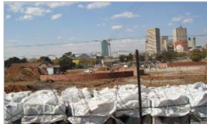
Figure 69. The same view in July 2009- Construction of Jazz Park funded by Tshwane Municipality (Author, 2009)
