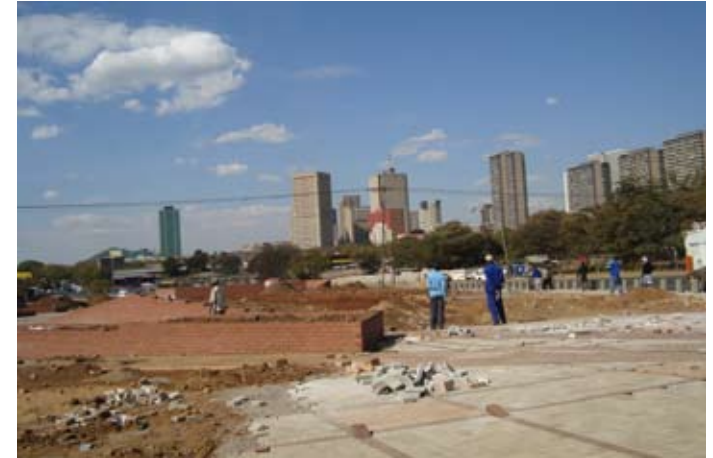
Figure 88. Looking East towards Pretoria CBD. Jazz Park under construction (Author, July 2009)
