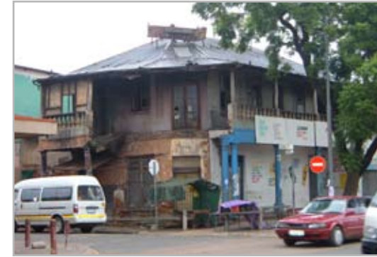
Figure 14. Dilapidated Building (Author, 2009)
