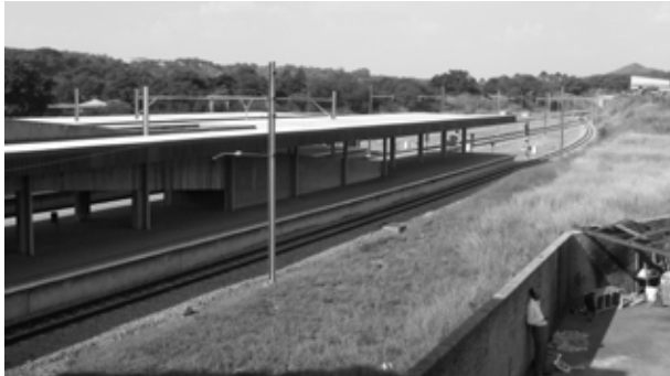
FIG 2.1_Belle Ombre metro rail station
