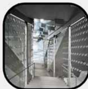
Fig 7.159 An example of a skylight. ( www.inhabitat.com )
