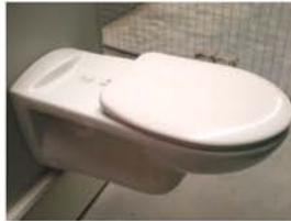
wall hung disabled WC
