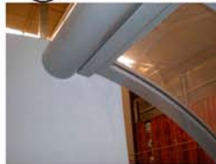
Silver PPC steel sections, and clear polycarbonate
