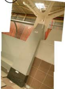
polished black granite skirting tiles, painted grey, steelwork painted white
