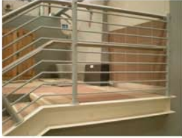
grey painted GM steel balustrade with stainless steel handrail at high low heights
