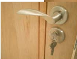
brushed stainless steel ironmongery with disabled accessible latch (top)
