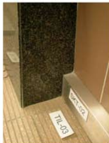
polished black granite skirting tiles, painted grey, steelwork painted white
