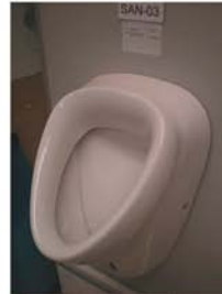
urinal and flush plates
