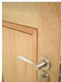
wooden doors with brushed stainless steel ironmongery and double rebate door detail
