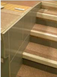
contrasting colour nosing for visibility, return on handrail for accessibility, grip tread
