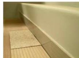
profiled concrete bench, painted chalk white with polished ceramic tile skirting
