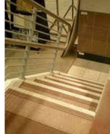
contrasting colour nosing for visibility, return on handrail for accessibility, grip tread
