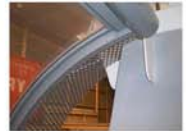
Silver PPC steel sections, and clear polycarbonate
