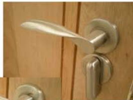
wooden doors with brushed stainless steel ironmongery and double rebate door detail
