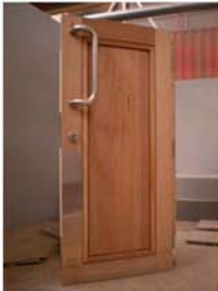
wooden doors with brushed stainless steel ironmongery and double rebate door detail
