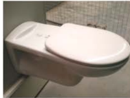
wall hung disabled WC
