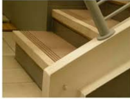
grey painted GM steel balustrade with stainless steel handrail at high low heights
