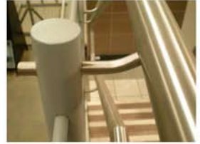
grey painted GM steel balustrade with stainless steel handrail at high low heights
