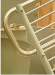
contrasting colour nosing for visibility, return on handrail for accessibility, grip tread
