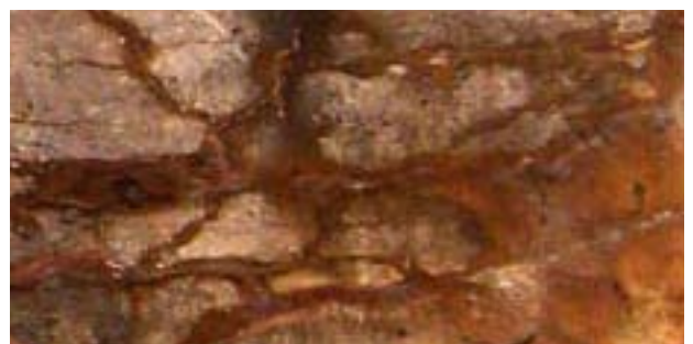
Figure 7.08 Texture of existing concrete structures
