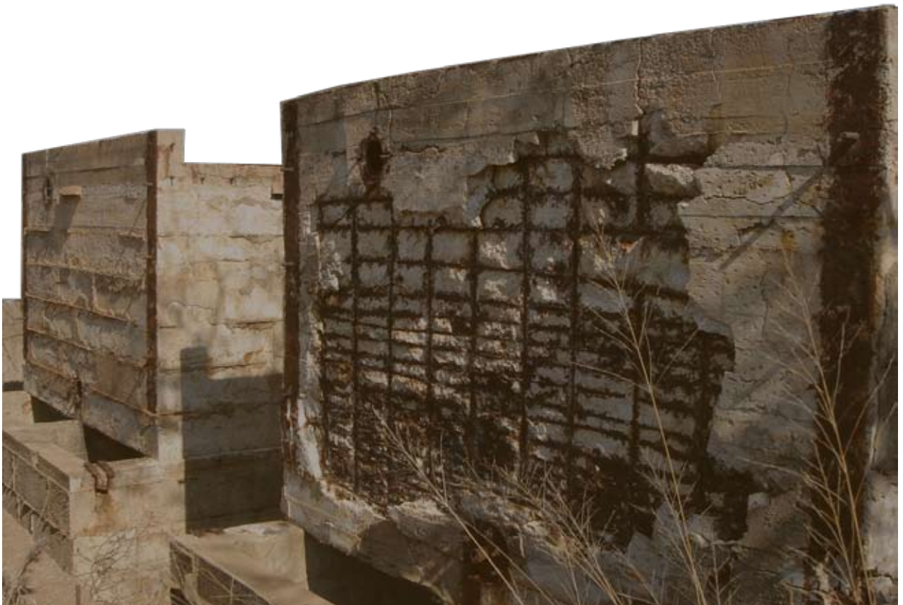
Figure 7.02 Existing corroding reinforced concrete structures. It is suspected that these structures were used as storage tanks for the water and brine that was pumped from the crater floor. [August 2009]
