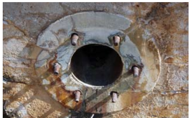
Figure 7.07 Materiality of existing concrete structures
