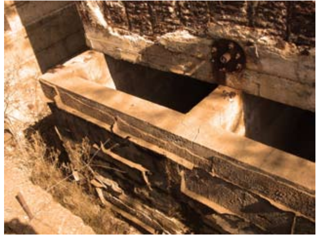
Figure 5.22 Reinforced concrete storage tanks [March 2009]
