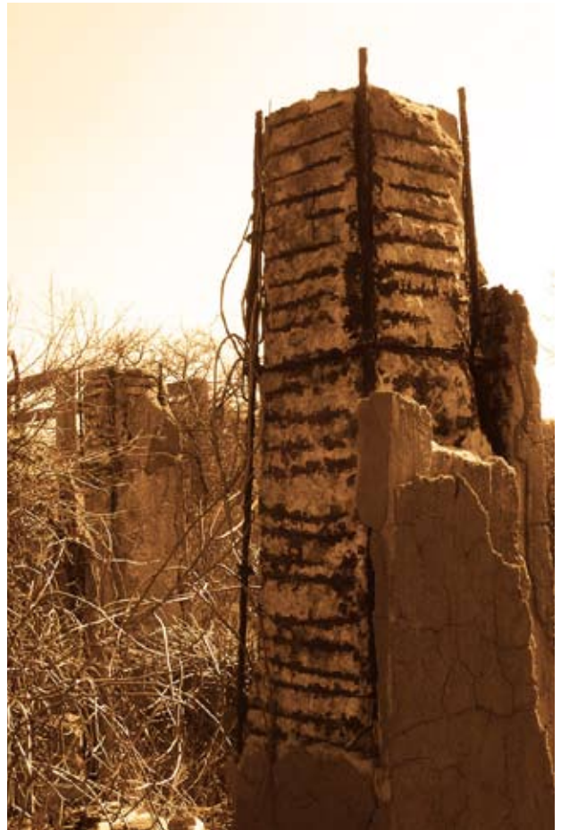
Figure 5.23 Reinforced concrete column structure [March 2009]
