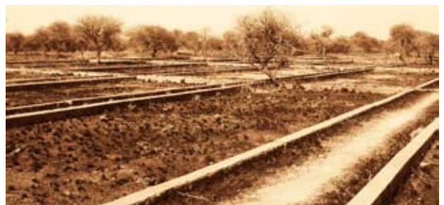
Figure 5.24 Foundations of historic warming ponds [August 2009]
