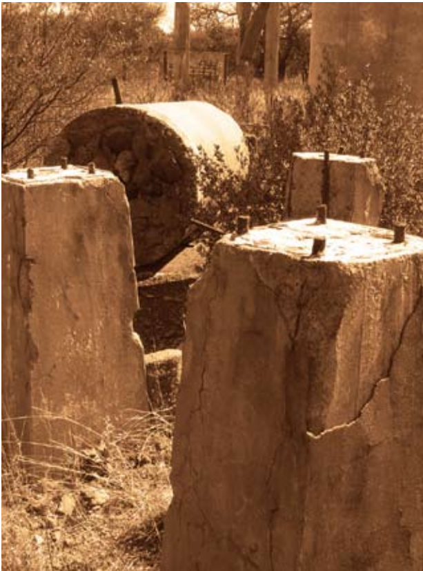
Figure 5.21 Reinforced concrete elements [March 2009]
