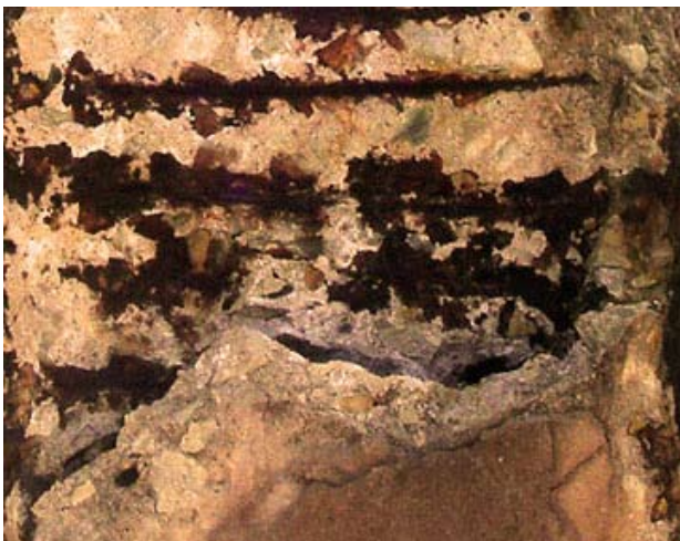
Figure 5.05 Corroded reinforced concrete storage tank structure [March 2009]
