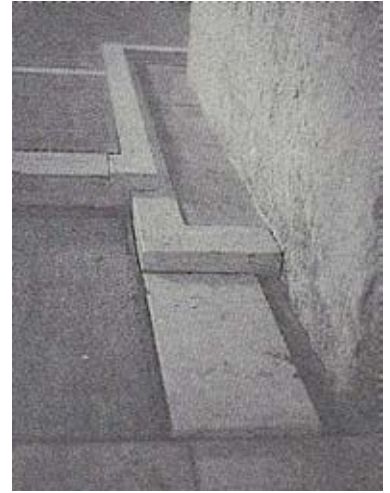
Figure 4.10 Detail of the paving edge at the threshold between the entrance room and the sculpture gallery. A tiny cascade of levels formed from white Prun stone. [Murphy, 1999:49]
