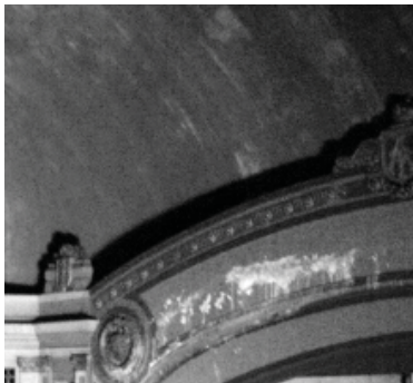
Figure 9.2 Dome rising from rear of proscenium
