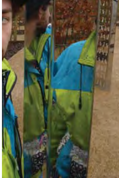
Figure 9.16 Stainless steel used for finish on columns, either brushed or polished
