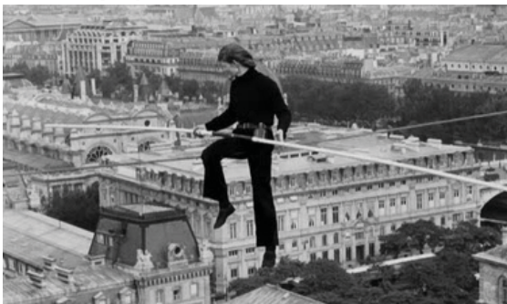
Figure 6.20 Still image of Philippe Petit crossing between towers of Notre-Dame, Paris
