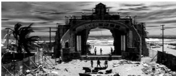
Figure 6.13 Sycamore Grove Theatre abandoned proscenium.
