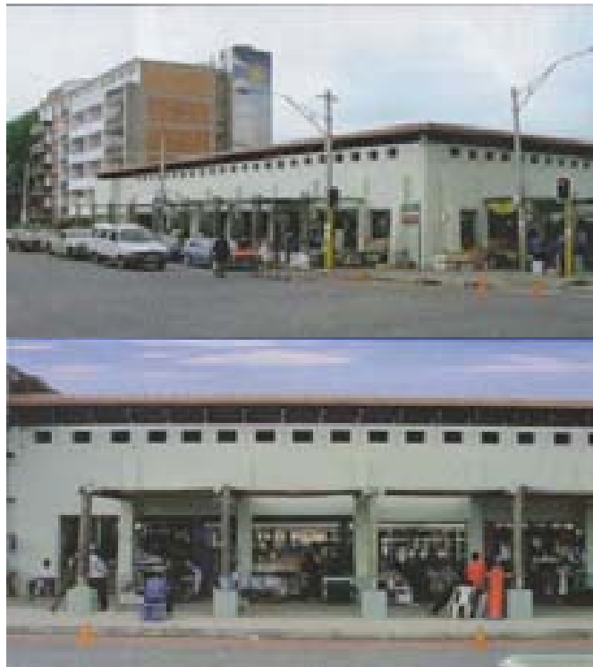
(Figure 118 & 119) Exterior photograph of building (Hansen, L. pp 44–45).
