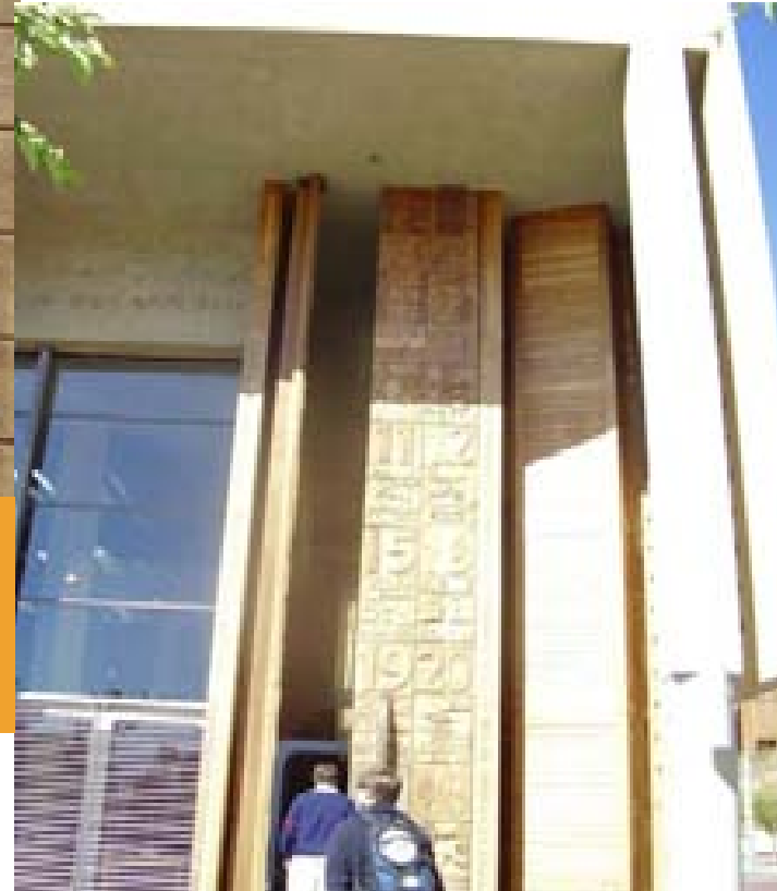
(Figure 107) Exterior showing signage that is placed on the front façade of the building (University of KZN field trip, class of 2005).
