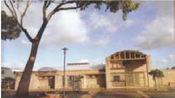
(Figure 126) Exterior photograph of building (Murray, 2008).
