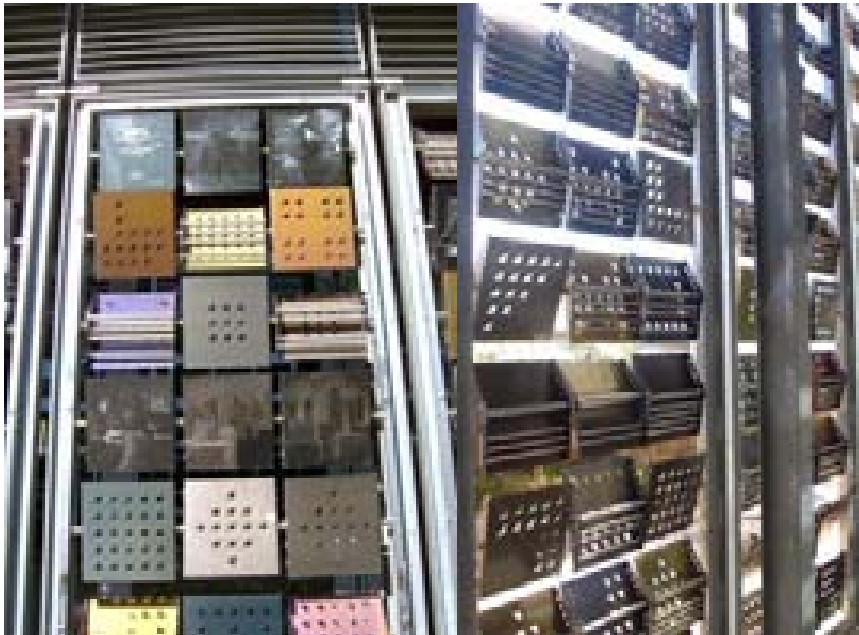
(Figure 108) Exterior detailing of façade panels. These detailed tip-up screens are conceived by Andrew Verster and are installed on the west façade (University of KZN field trip, class of 2005).
