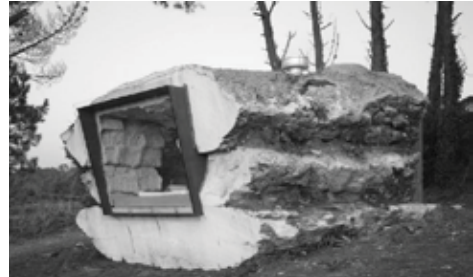
_9.6 The La Trufa concrete edge, cut with a 1800 mm diamond saw blade.
