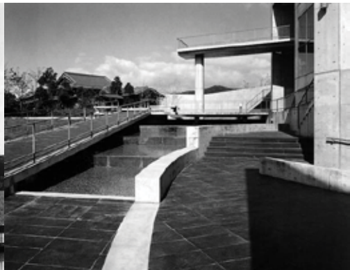
_4.8 Ramp across the pond
